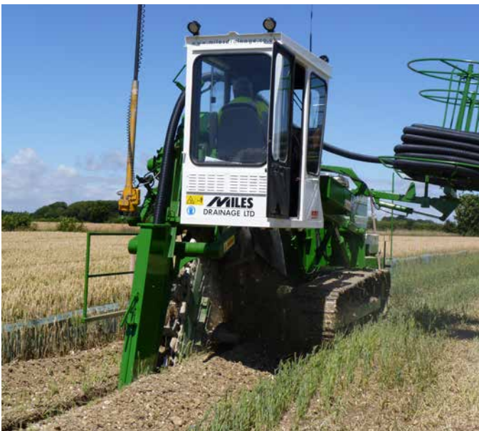
Figure 31. Installing land drains with laser gradient control
