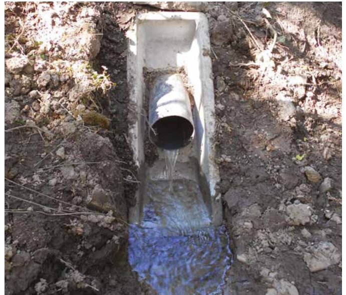
Figure 38. Precast concrete headwall (type K)
