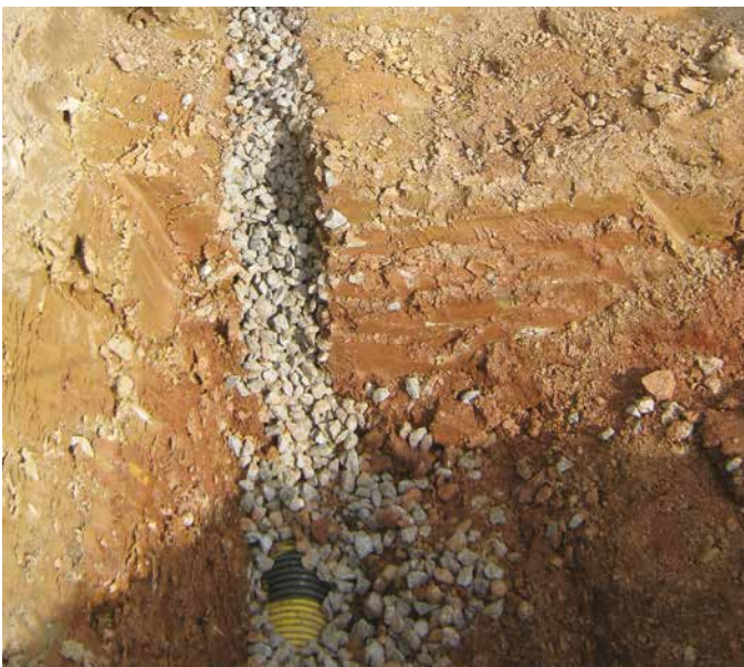
Figure 37. Washed gravel permeable fill over drain
