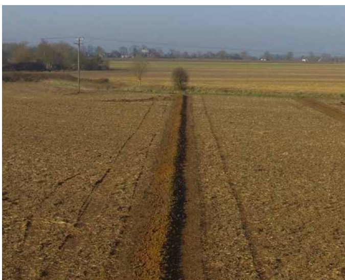
Figure 29. Recently installed drains
