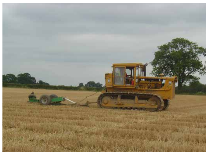
Figure 30. Installing mole drains
