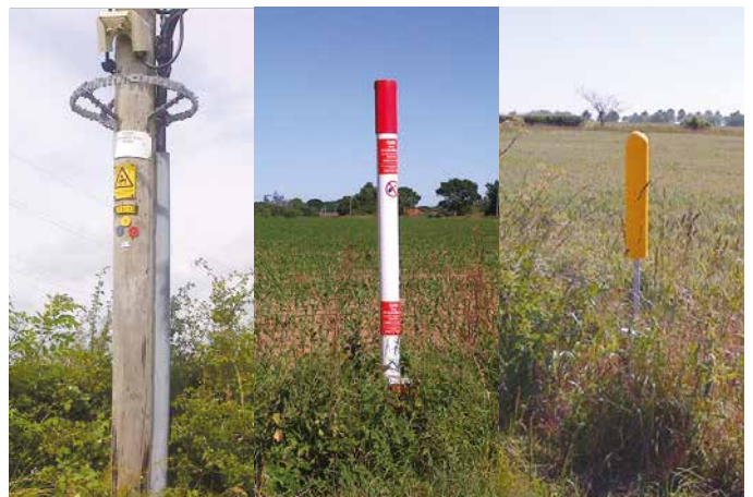
Figure 18. Signs indicating potential underground hazards
