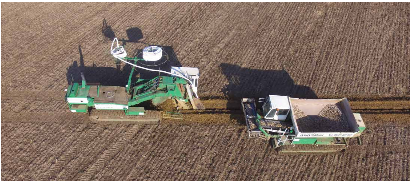
Figure 28. Installing land drains and stone backfill
